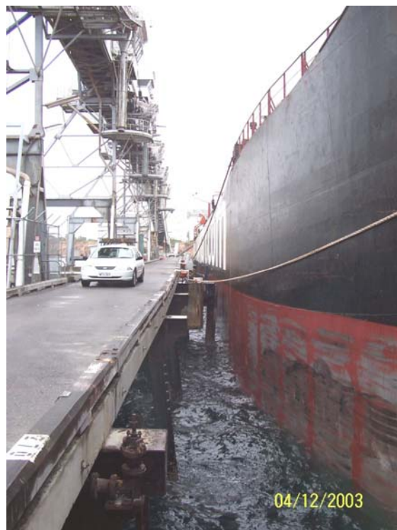
Above the first vessel in early December 2003 to use the first three new fenders and associated structures at Port Giles.
