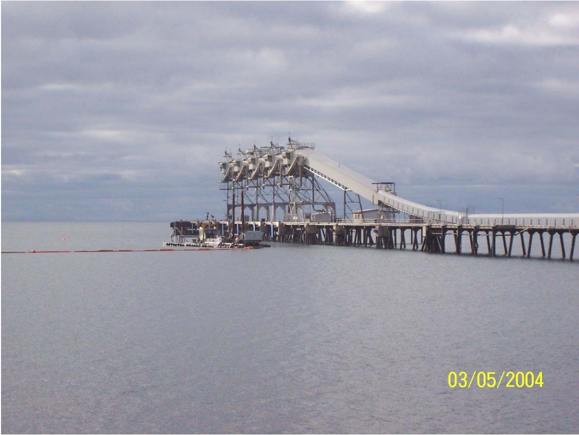
Dredge "Kikulu" at Port Giles
