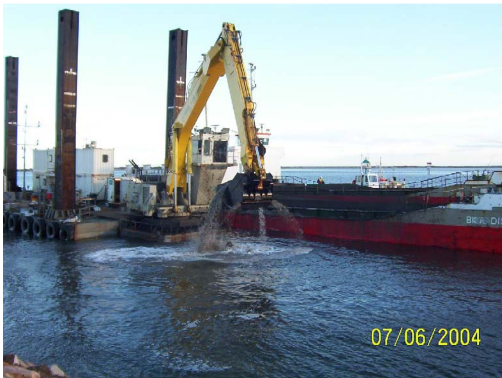
Dredge “Storcken” at work at Berth 8
