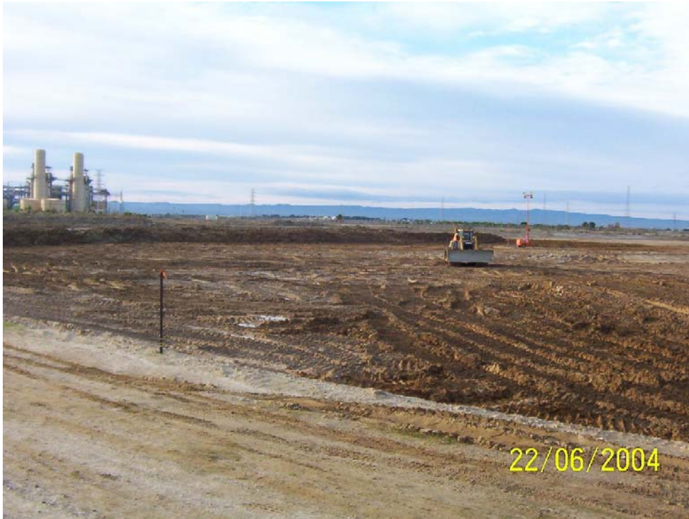
Dredged material being used as fill on adjacent land
